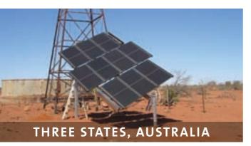
Submersible solar powered pumps such as the Grundfos SQFlex are becoming a highly viable alternative in outback Australia.
