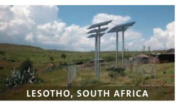
Five solar panels are utilised in the Grundfos SQFlex Combi solution in Mafeteng Mountains
